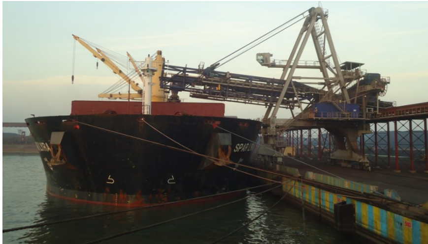
Ship Loader, Reclaimers
