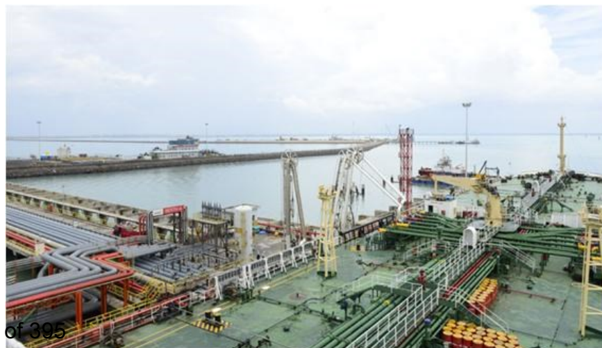
Jetty With Loading arms in operation
