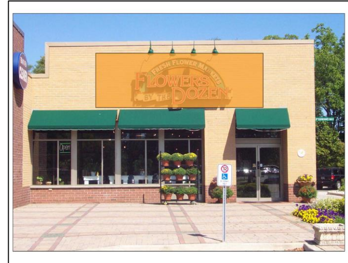
20% of Building Facade
