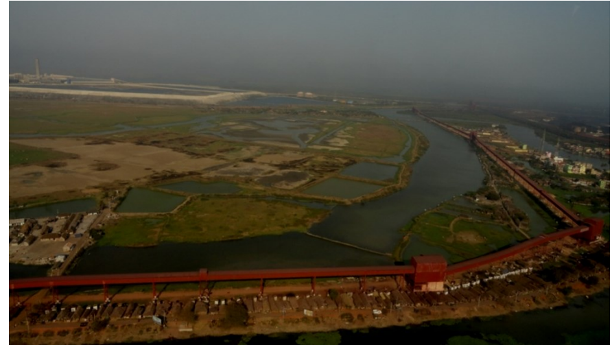
11 km long high capacity conveyor system
